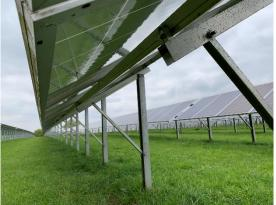
12.1.10. The PV Modules are then attached to the Mounting Structure to form the PV Table. This stage is also non-intrusive to the ground and the only impact is from vehicular access, carrying in the panels. It can be seen that if ground conditions are suitable, there is no damage. The photograph below simply shows bruised grass from the passage of vehicles.
