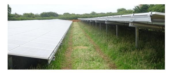
12.1.11. The cabling along the length of the PV Tables is hung underneath the PV Modules (out of the reach of sheep) and then, at the end of a row, it goes underground, as shown below.
