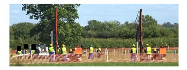
12.1.7. The details vary slightly between panel manufacturers, but the Mounting Structures (for Fixed South Facing) will have a taller and shorter stanchion, as shown below. The lack of damage or disturbance to the grassland and ground conditions from this operation is evident in this photograph.
