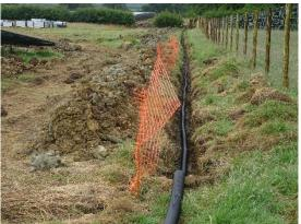
12.1.13. The installation of cables is one of the few operations that involves digging whereby the soil structure could potentially be affected. The trenches are always narrow, but soil is required to be dug up to install the cable, as is
