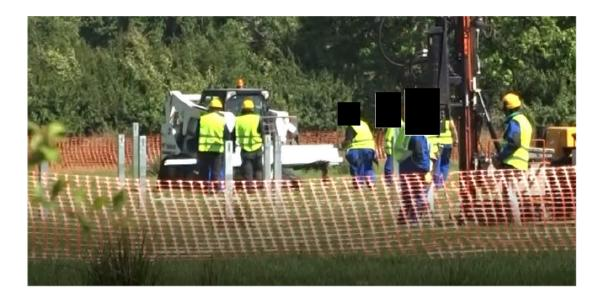
12.1.5. A team then arrives to knock the stanchions / legs in. From operations we have observed it takes a little over a minute per pole to knock the pole into the ground and move the machine to the next pole<sup>1</sup>. This operation is shown in the photograph below. This was inserting legs into a clay soil, but the deep stoneless soil at the Order limits will be similar.
